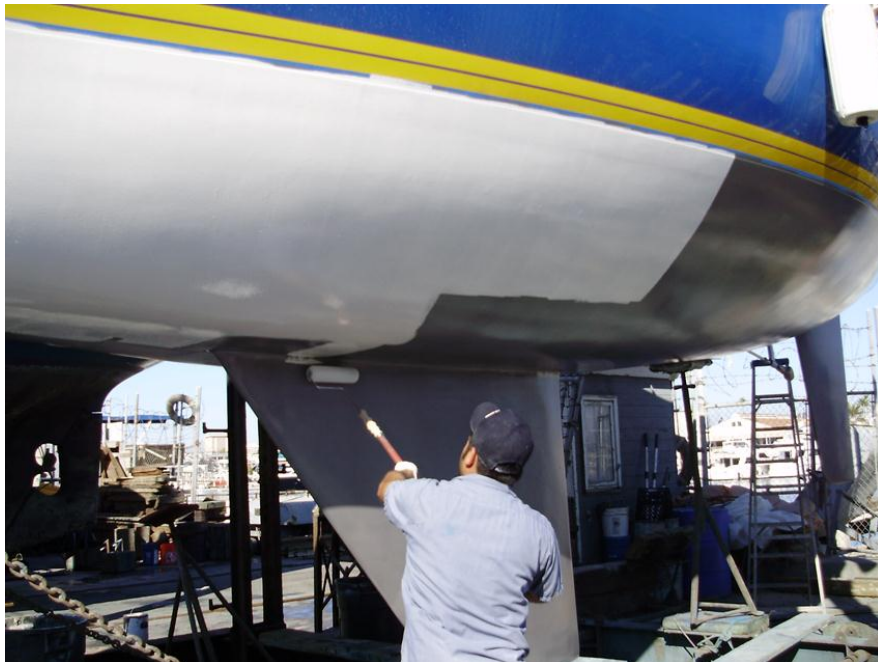
Figure 5-30. Painter Applying Sealer
