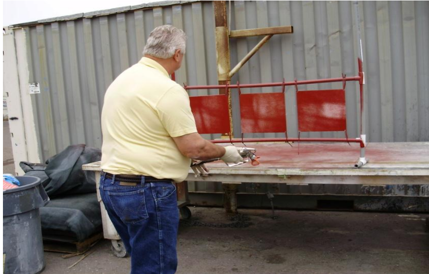
Figure 3-3. Supplier Spray Painting Panels
