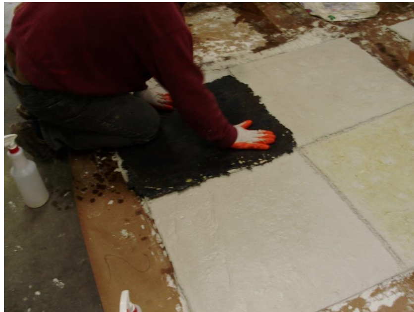
Figure 2-10 Placing Stamp Mat for Release Agent Testing at Multicoat
