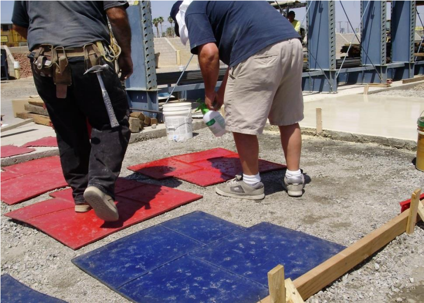
Figure 2-2 Spraying Stamp Mat with Release Agent
