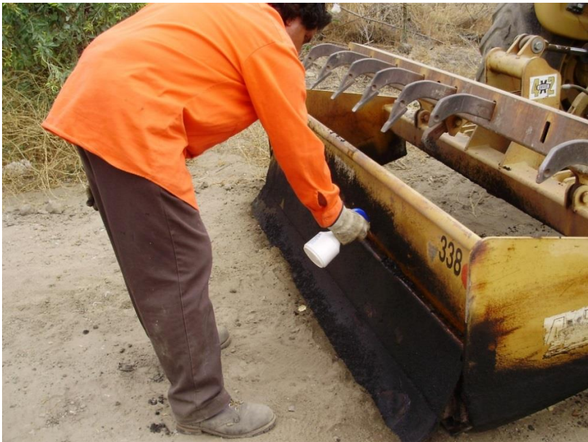
Figure 2-22 Spraying Release Agent on Tractor Scoop
