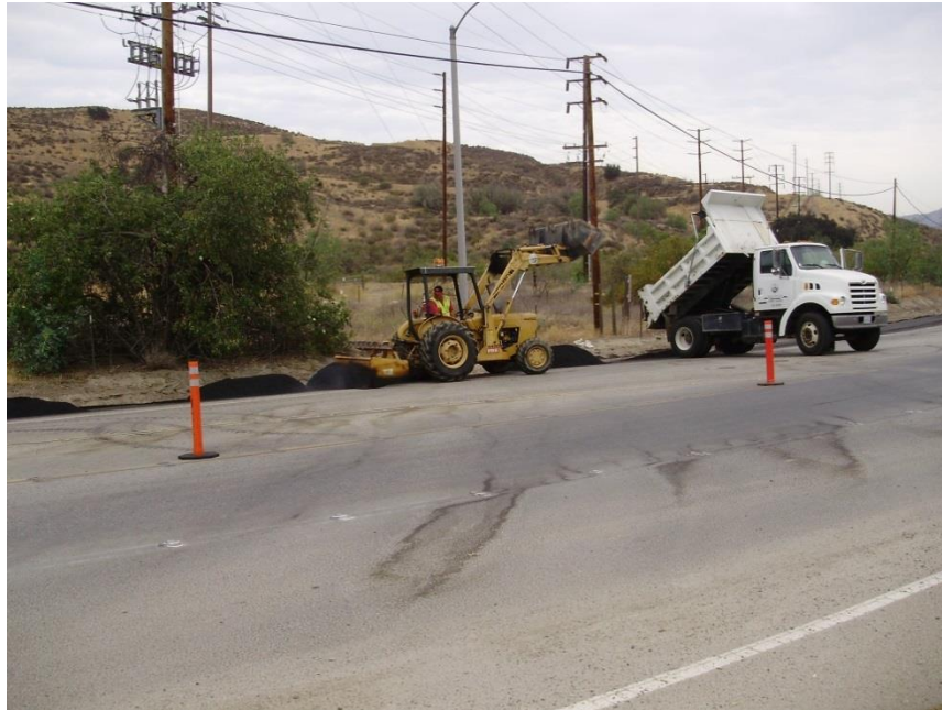
Figure 2-17 Truck Dumping Asphalt for Application in Simi Valley
