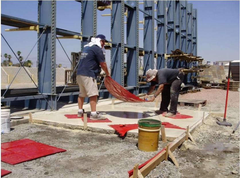
Figure 2-3 Laying Stamp Mat on Concrete
