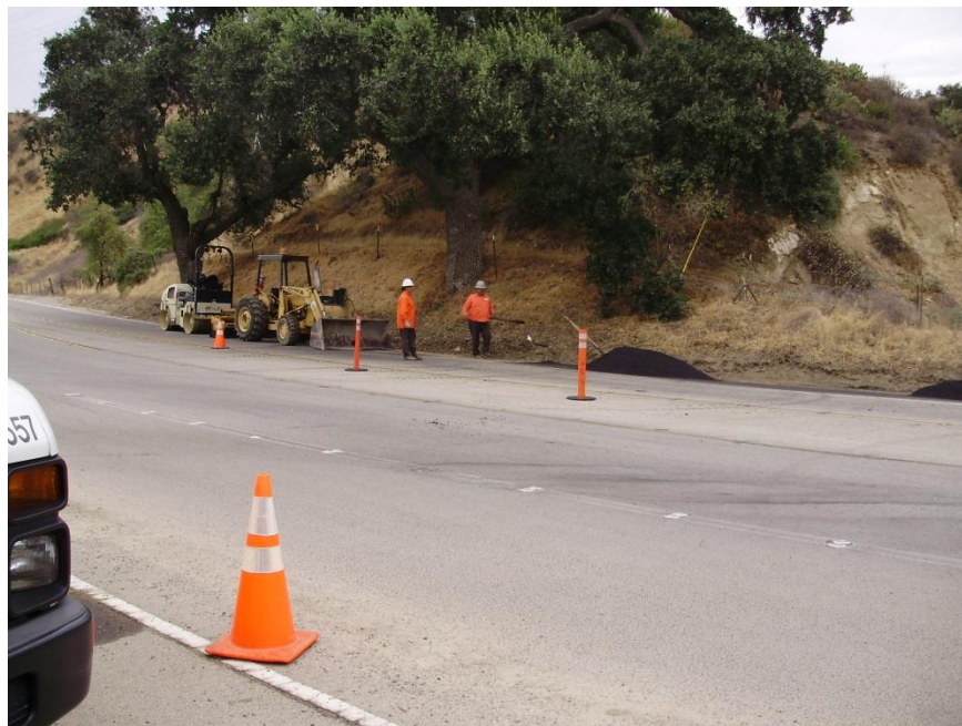
Figure 2-16 Simi Valley Workers Applying Asphalt
