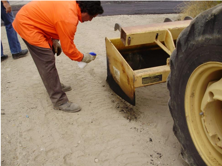
Figure 2-21 Spraying Release Agent on Tractor
