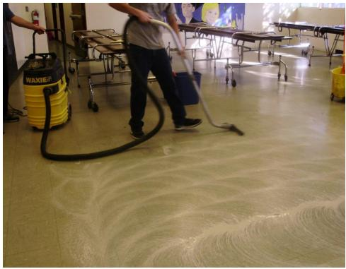
Figure 2-3. Wet Vacuum Handling Residue
