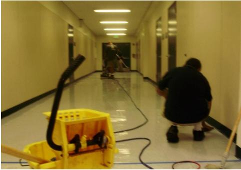
Figure 3-2. Workers Applying Vinyl Seal Coating
