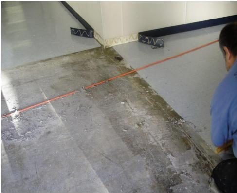
Figure 4-3. Workers Installing EcoPure Flooring
