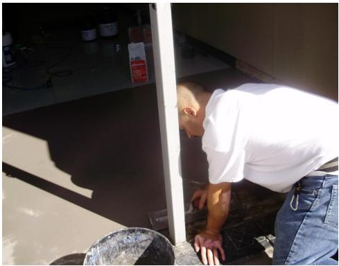
Figure 4-1. Workers Installing Optima IQ Flooring.
