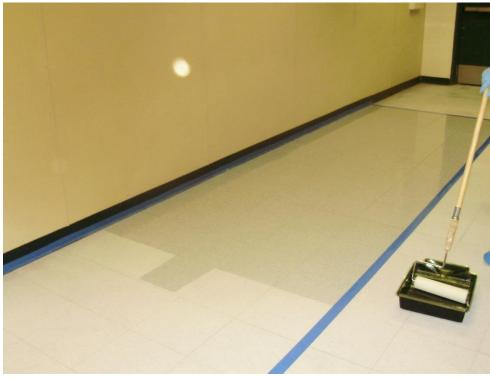
Figure 3-8. Workers Applying UV Coating
