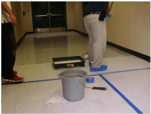
Figure 3-5. Workers Applying Polyurethane Coating
