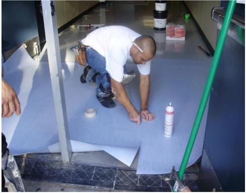
Figure 4-2. Another View of Workers Installing Optima IQ Flooring
