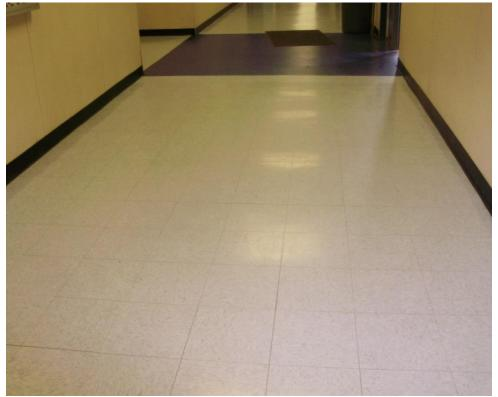
Figure 3-7. Polyurethane Coating at End of School Year
