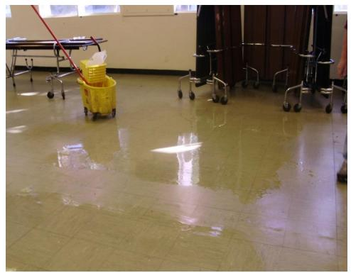
Figure 2-1. Stripper Applied to Floor
