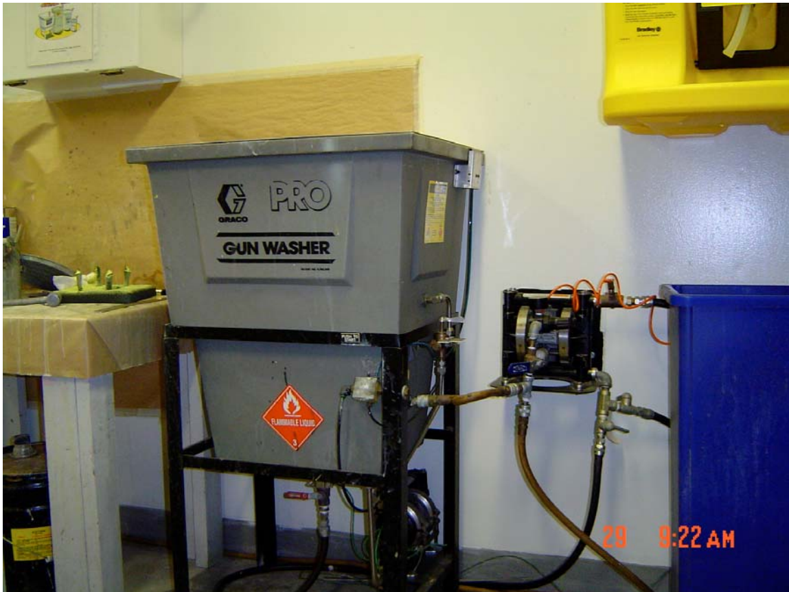
Figure 3-1. Spray Gun Cleaning System at Hydro-Aire
