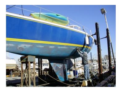
A primer is applied to these spots and then a copper topcoat is applied over the prepared hull surface. In some cases, the hull paint is stripped from the boat, often using hand sanding methods. The hand sanding dust from surface preparation or stripping is the second waste stream that contains copper. Some boatyards are starting to use abrasive blasting media to strip boats and the spent media is the third waste stream that contains copper.
