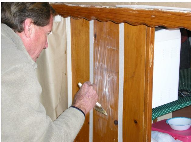
IRTA also evaluated alternative stripping methods for removing the copper antifouling paint from boat hulls. In this project, sponsored by EPA Region IX and DTSC, chemical strippers are not the best option for stripping the hull. The best alternative options are to hand sand the old coating or to remove it with a blasting technology. Three different blasting systems were evaluated and the cost of using all the technologies was compared.
