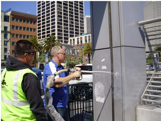
The two different systems can complement each other. The dry ice blasting system is less aggressive than the crushed recycled glass system. The systems can be used together to clean graffiti from a variety of surfaces including lamp posts, concrete walls and parts of various kinds, metal structures and parts and porous surfaces like granite
