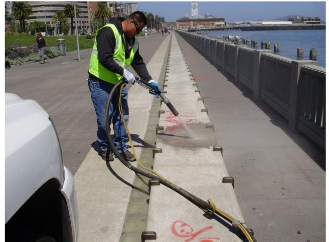
The systems performed well on metal powder coated substrates that are used as supports and for fabricated chairs on a dock on the Embarcadero that is owned and maintained by the Port. The crushed recycled glass system was very effective in removing old faded graffiti from concrete sidewalks. Other systems had not been able to remove this embedded graffiti.
