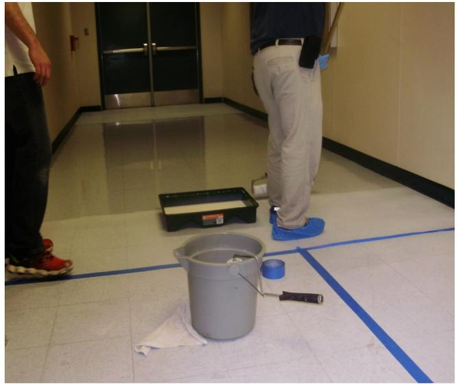
The vinyl seal is likely to last a shorter time than the polyurethane coating. The UV curable coating is likely to last even longer before another application is needed. These coatings do not require wax to be applied and the maintenance regime is simply to clean them with plain water or a neutral water-based cleaning solution on a regular basis. The polyurethane and UV curable coatings have a very high gloss and the vinyl seal has a lower gloss.
