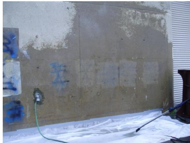
Figure 4-6. Concrete wall after rinsing
