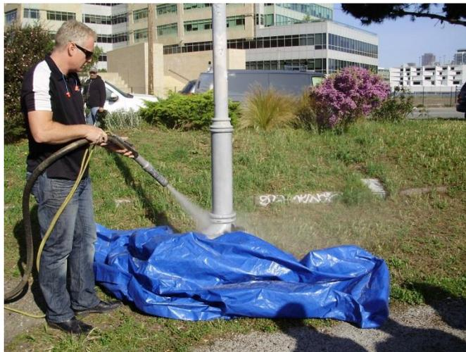
Figure 3-3. Blasting system removing graffiti from lamppost
