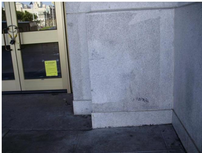
Figure 2-9. Building with graffiti resistant coating showing shadowing
