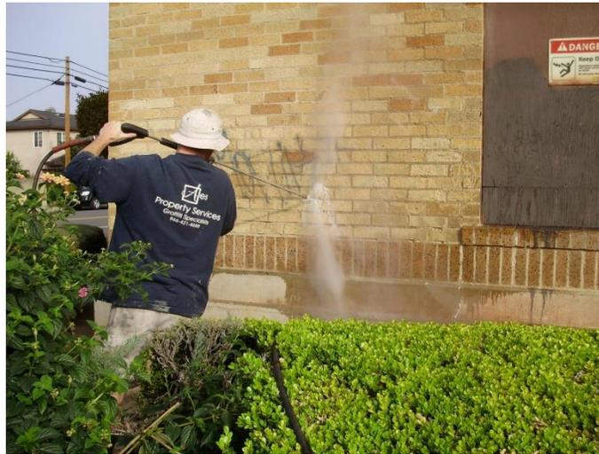
Figure 2-4. Contractor using soda blasting system
