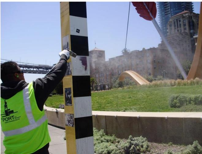
Figure 3-15. Glass blasting system removing sticker from pole
