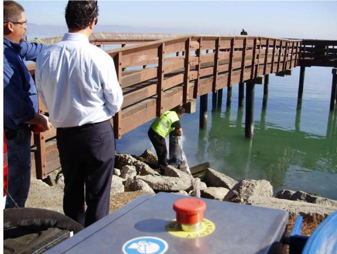
Figure 3-16. Dry ice blasting system removing graffiti from pier
