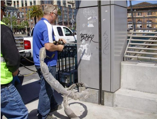
Figure 3-8. Dry ice blasting system removing graffiti from post
